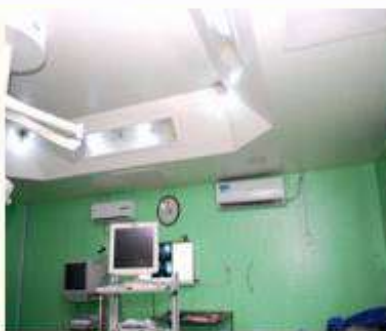
Renovated roof with lightning and monitor
